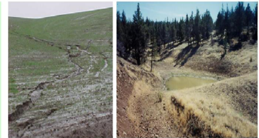
To reduce sediment (left) from entering tributaries in the Pine Hollow watershed, sediment control basins (right) have been created in the uplands. (Photographs: Courtesy of the Sherman County Soil and Water Conservation District.)
