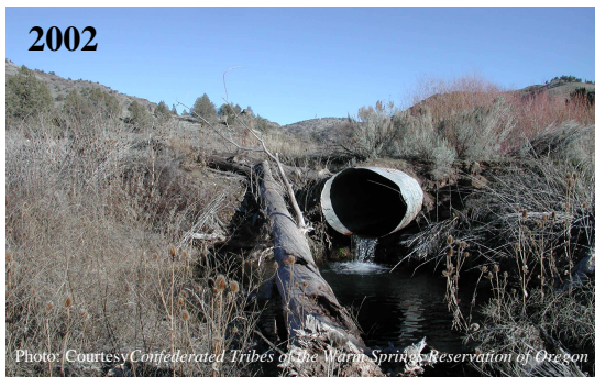
Working with the Wheeler County Soil and Water Conservation District, the Confederated Tribes of the Warm Springs Reservation of Oregon removed the culvert in the above photo (left) that was functioning as a barrier to fish passage.
