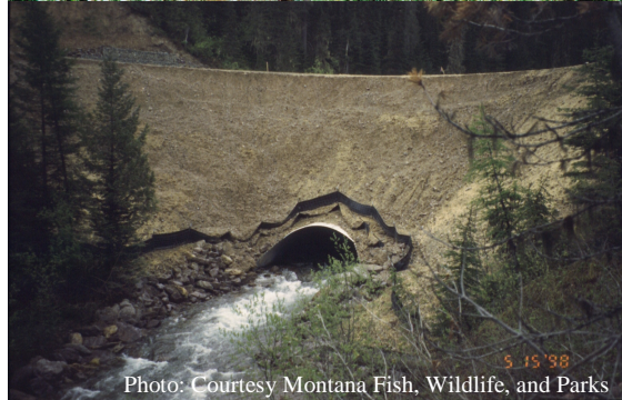
Prior to replacement (upper photo), the Felix Creek culvert prevented fish from moving upstream.
