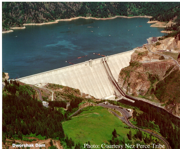
Dworshak Dam, Idaho
