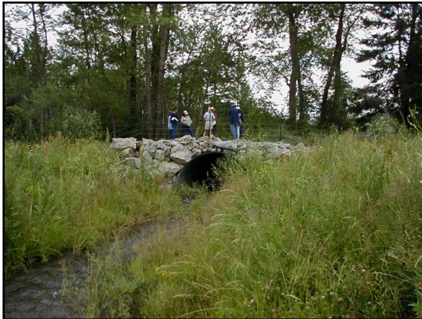
Open arch culvert and new approach channel on Ronan Creek.
