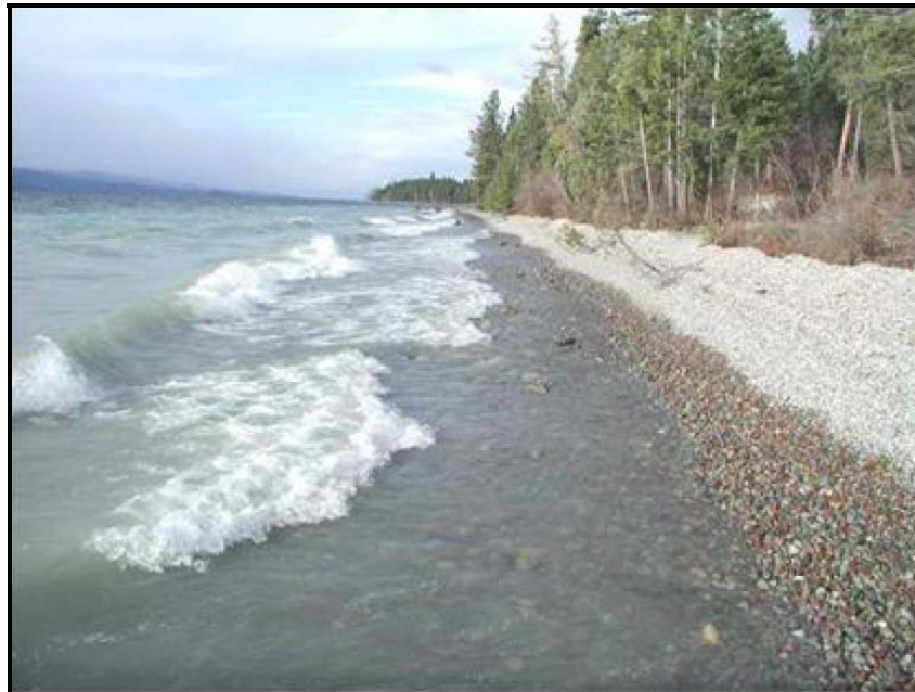
Same beach after restoration, illustrating energy dissipation of waves as they approach the back-beach.
