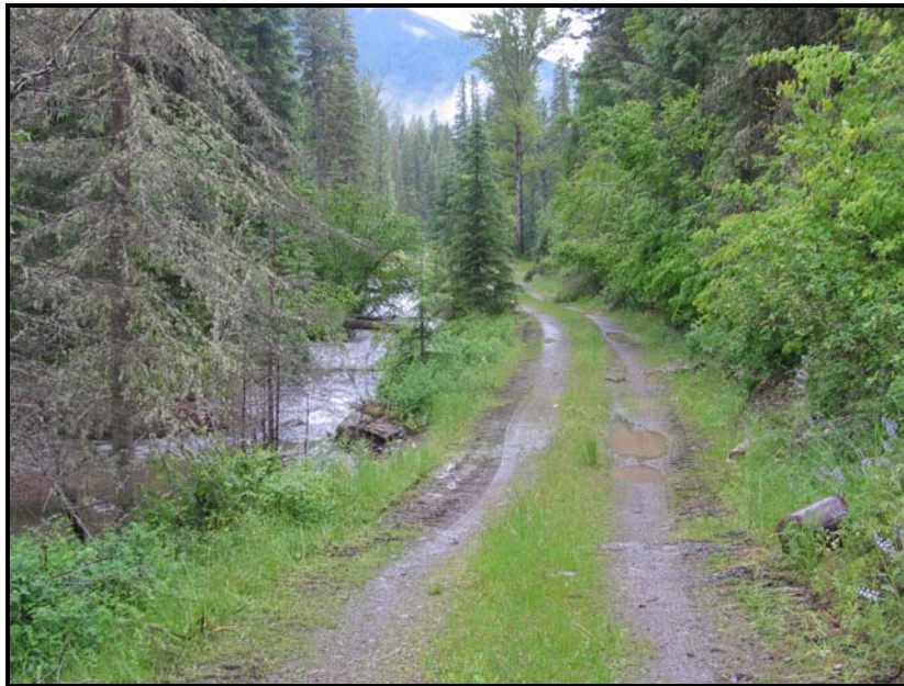
Road 3001 within the riparian area of the North Fork Jocko River, 2005.
