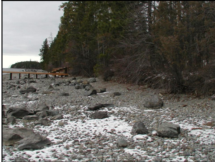
West-facing beach illustrating the eroding vertical bank.
