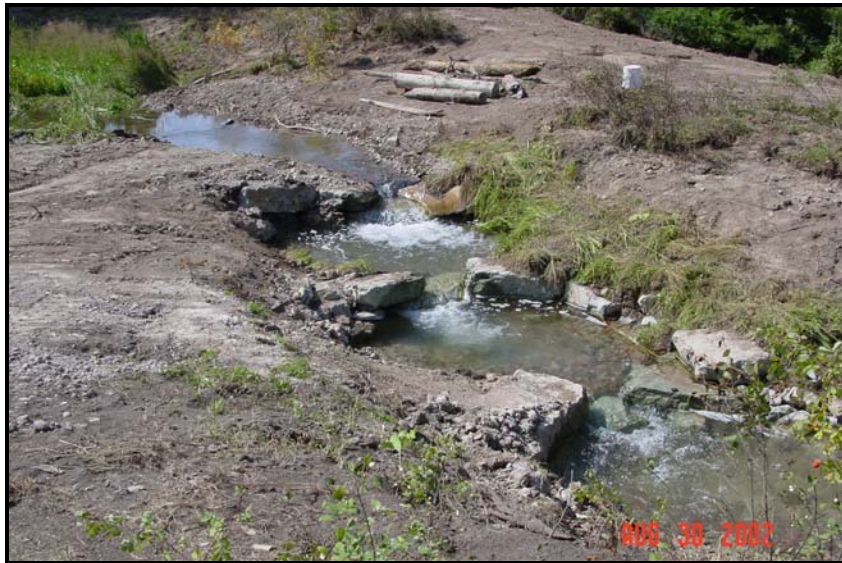
Completion of construction phase of rock weirs, August 2002.
