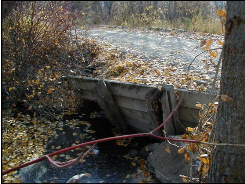
Ronan Creek crossing at Red Lake Road prior to reconstruction.
