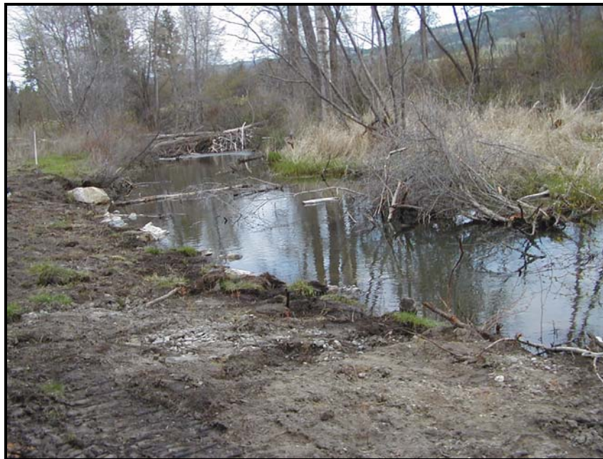
Bank of Dayton Creek after reshaping and armoring.
