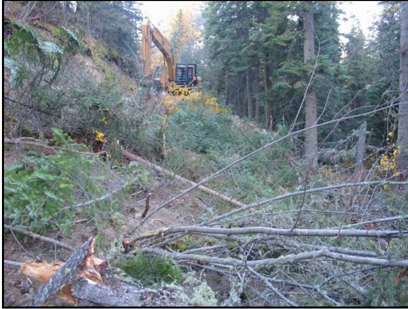
Same site during recontouring and slash covering.
